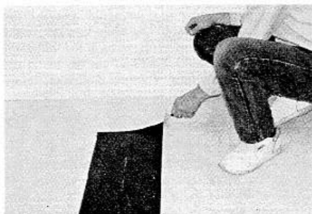
Removal of tile over subfloor joint.
