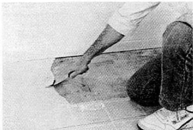
Scrape from remaining floor covering.
