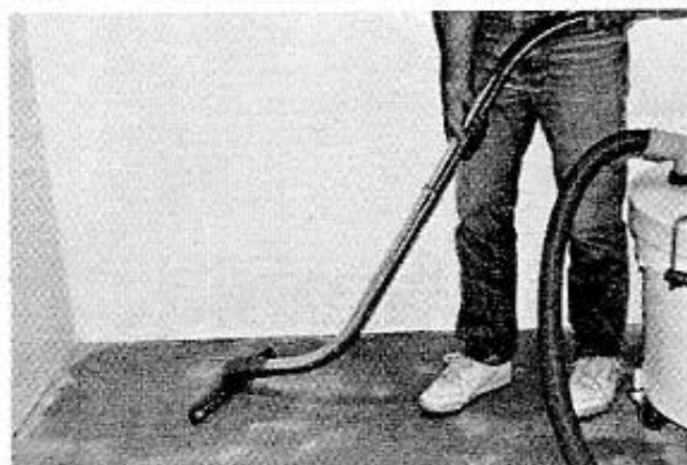
Vacuuming entire floor.
